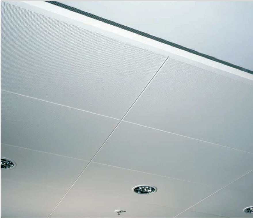
Clip-in and hook-on ceilings are also suitable for use in restricted void areas and with visible perimeter profiles when used as a ceiling island.
