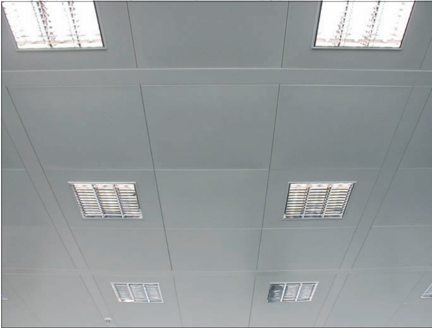
Cross bandrastrer ceiling with 9 panels per module.
