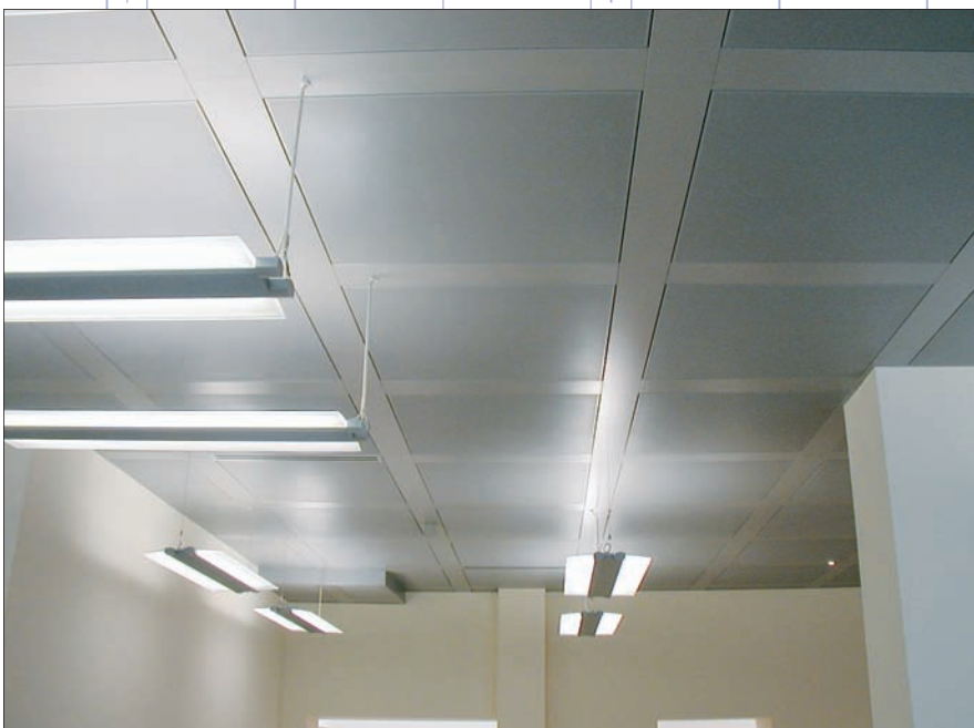
Cross bandrastrer ceiling with 1 panel per module.
